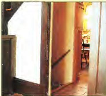
The entry to Mary's basement is in a high-traffic hallway. There's no door and no light—a perfect opportunity for kids to fall down the stairs. All stairwells must have sturdy doors.
